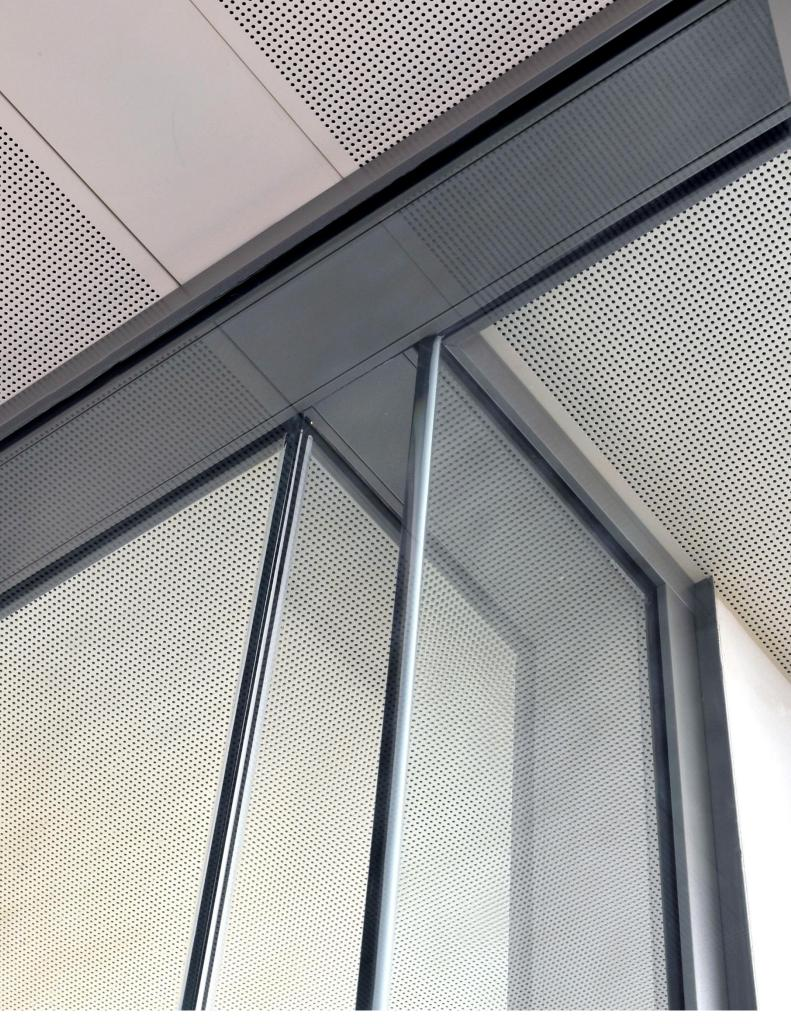
SAS System 8000 DG Three way head track junction detail
